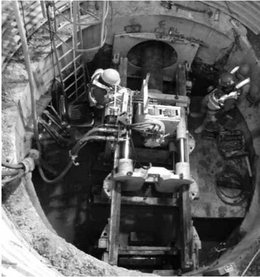
Jacking machine for pipe jacking
