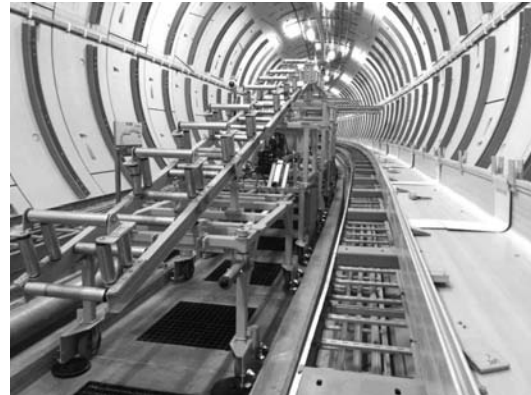
Cable pulling and laying machine
