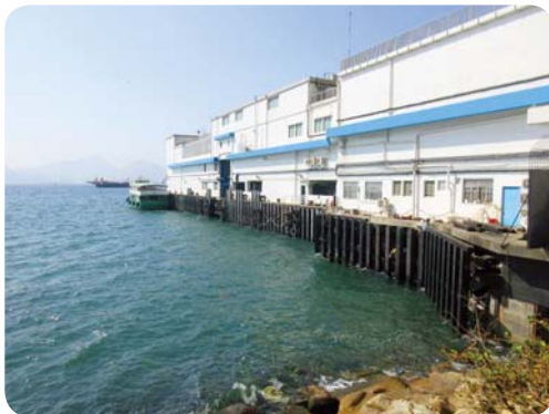
Civil Engineering and Development Department Maintenance Contract for Piers (2017-2022)
