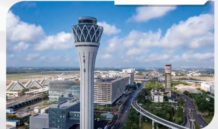
The civil works of the new tower was successfully completed and accepted. 新塔台土建工程順利通過竣工驗收。
