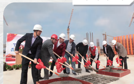
The positive and negative zero (正負零) in the central area of Terminal 2 and the steel structure in the corridor area were capped successfully. T2航站樓中心區正負零及指廊區鋼結構順利封頂。
