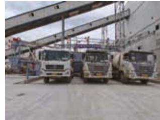
Separation of left materials and rinsing the inner side of tank on concrete mix truckers 剩料分離、刷罐
