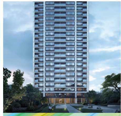
Hangzhou Lotus Mansion 杭州荷源府
