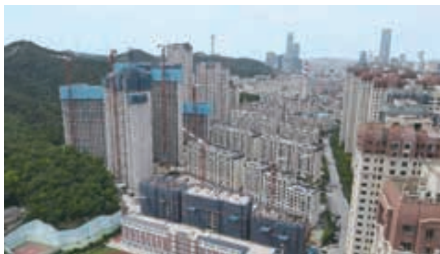
The construction site of the Dalian Glory of the City project
