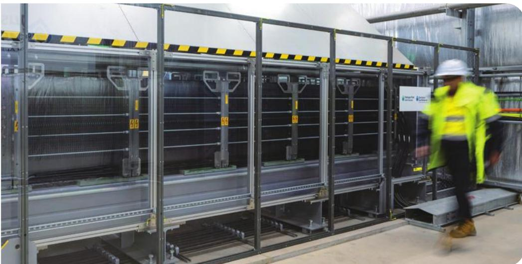
AGN's zero-emissions 1.25-MW electrolysis plant in South Australia creates green hydrogen and enables completely zero-carbon heating.
