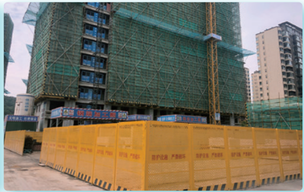
Examples of being equipped with protective facilities such as stable railings to protect workers' construction safety.
