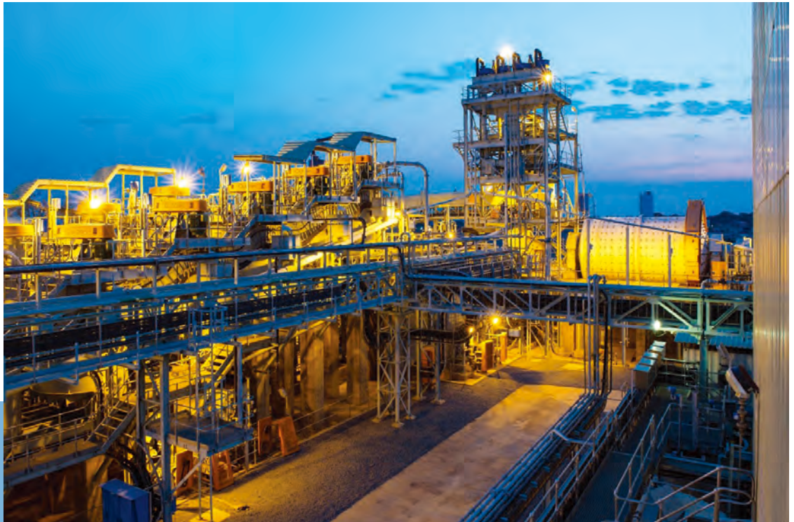
Kinsenda Processing Plant Kinsenda加工廠
