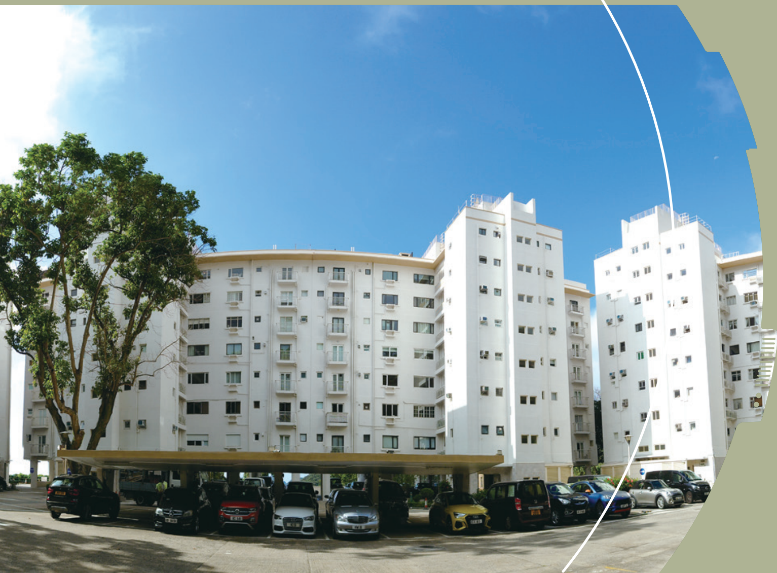
Renovation works at Carolina Gardens, The Peak 山頂嘉樂園之翻新工程
