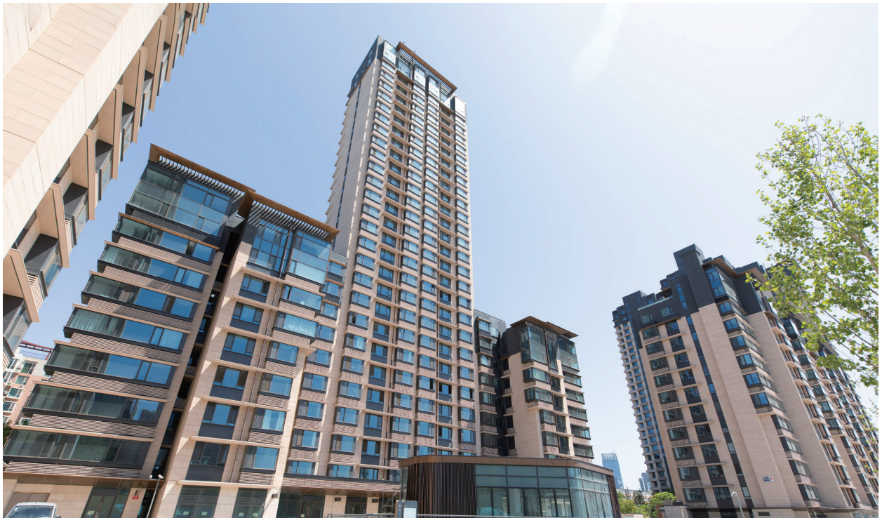
Development project "Capital Cove" in Tongzhou, Beijing
