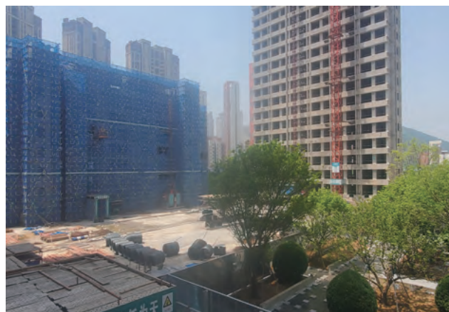
Construction Sites in Dalian
