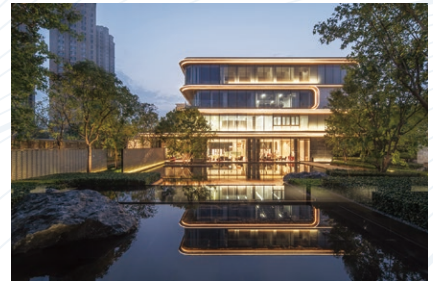
天津鉅悅公墅 Tianjin CIFI Park Mansion
