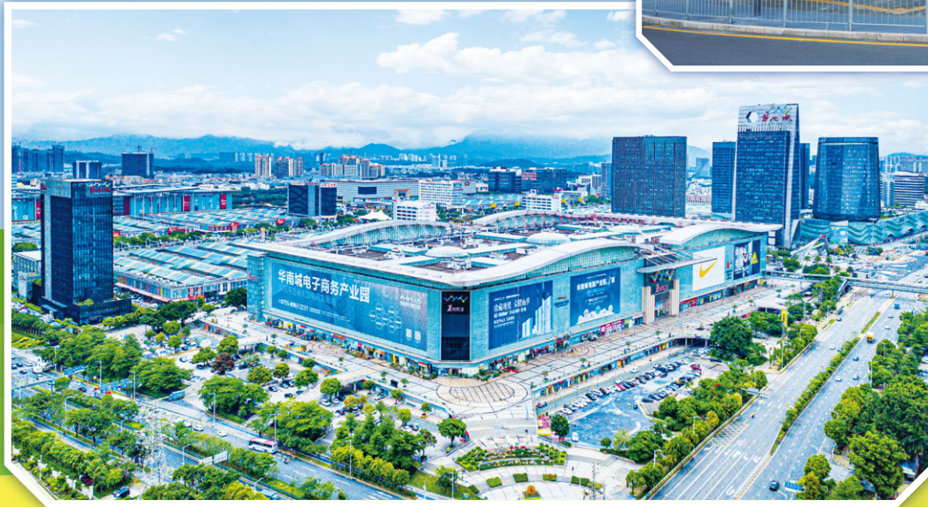
Trade Centres and Office Buildings in the Northwest of CSC Shenzhen 深圳華南城西北面 交易廣場及辦公樓群
