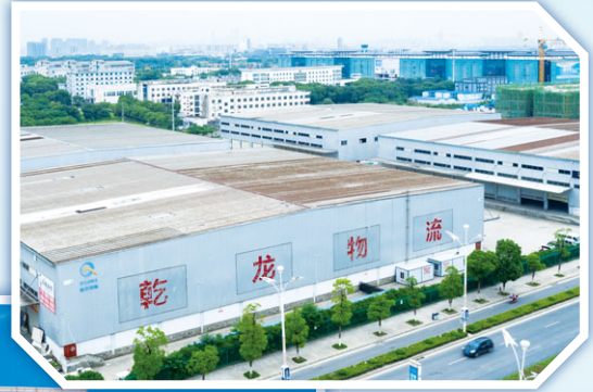
Qianlong Logistics Park in CSC Nanchang 南昌華南城的乾龍物流園
