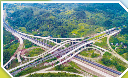
Yuqian Expressway Expansion Main Line in Chongqing 重慶的渝黔高速公路擴能主線
