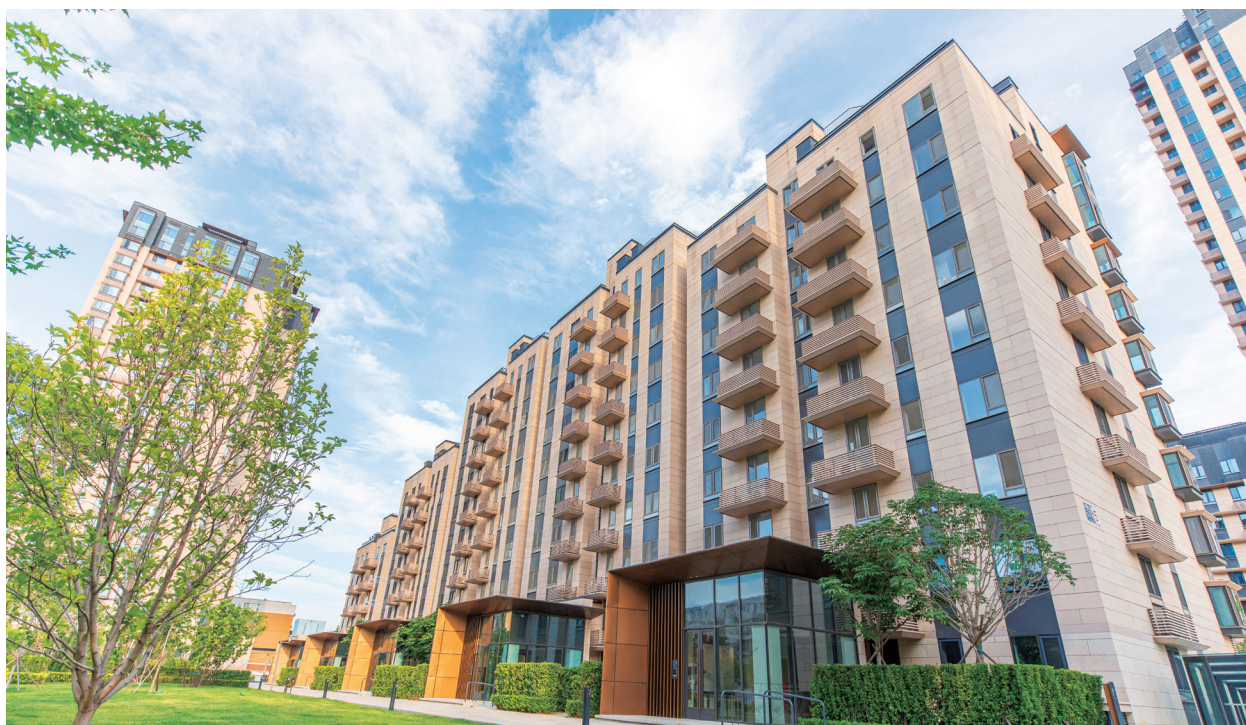
Development project “Capital Cove” in Tongzhou, Beijing
