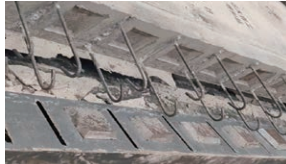
Picture 2: Shear key replacement for rough surface process
