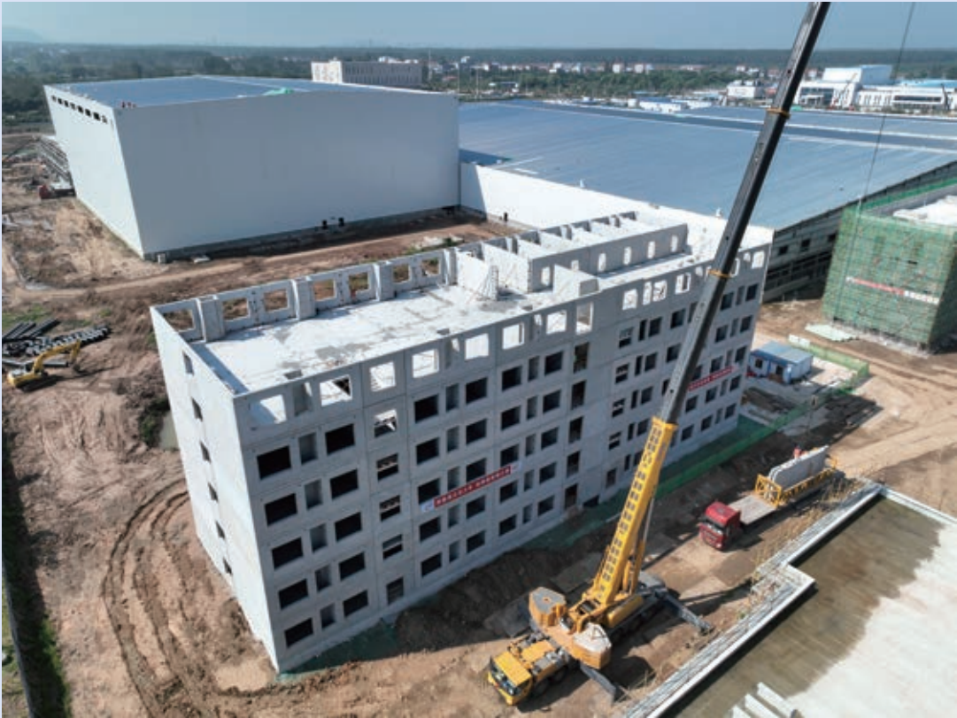
Picture 16: Yili's first green fully prefabricated digital construction project
