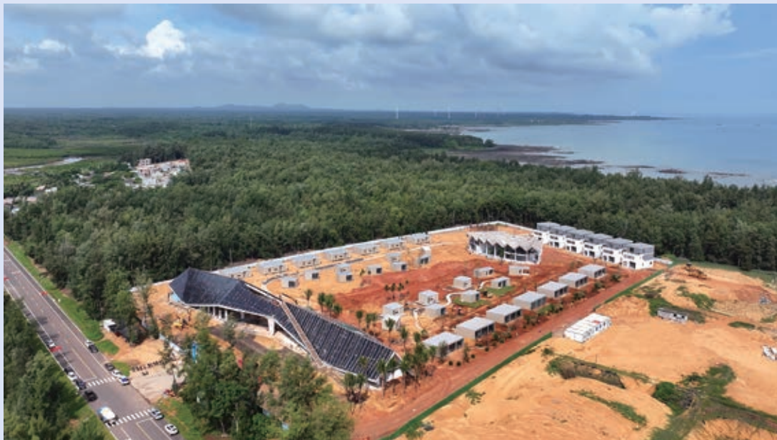
Picture 21: “Sunset Dan’er” Rest Stop project
