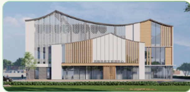
④ Energy centre construction service project
