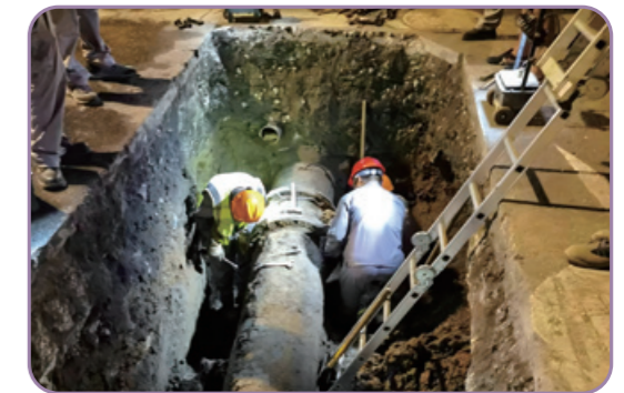
Gas pipelines renovation and construction sites
