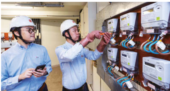
● Our engineers install smart meters to help customers understand and optimise their energy usage.
