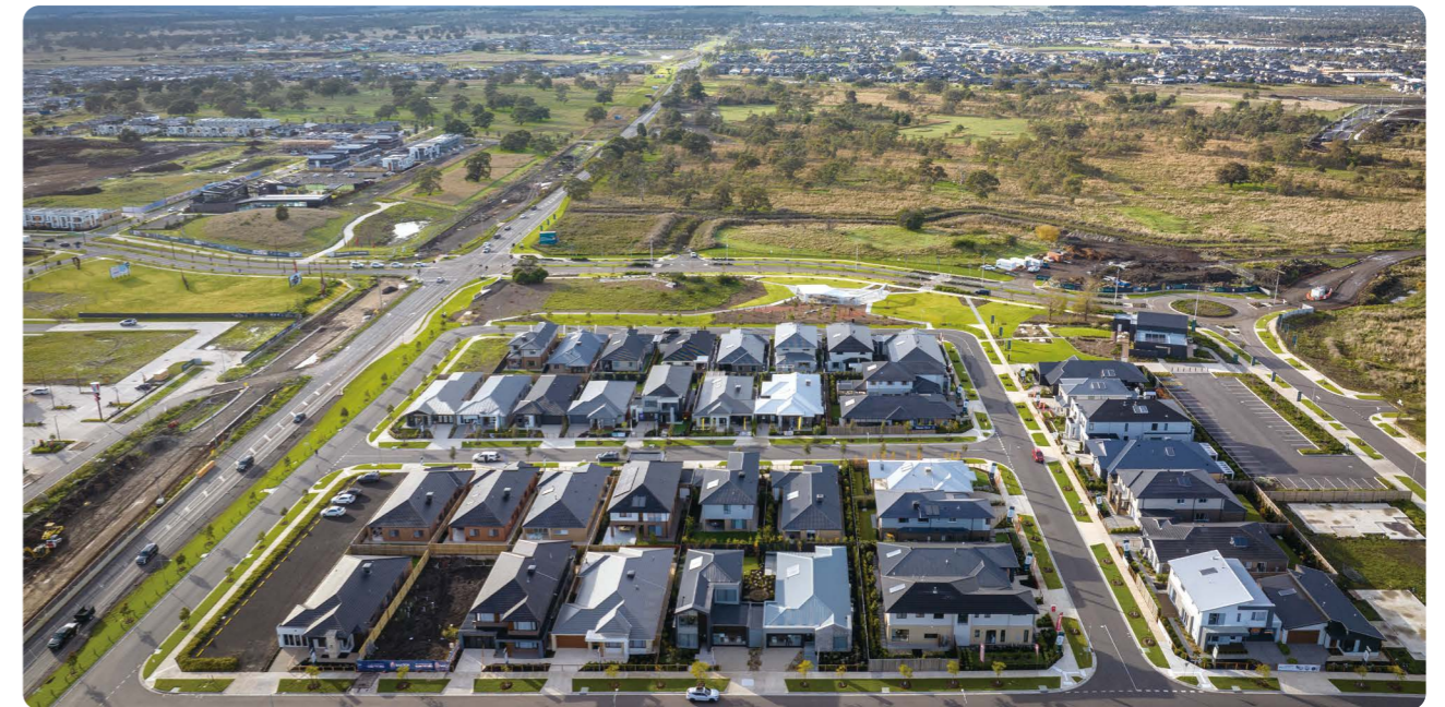
AGIG's HyHome, located at the Dennis Family Homes display centre in Wollert demonstrating future energy use where natural gas is replaced entirely by carbon-free hydrogen.
