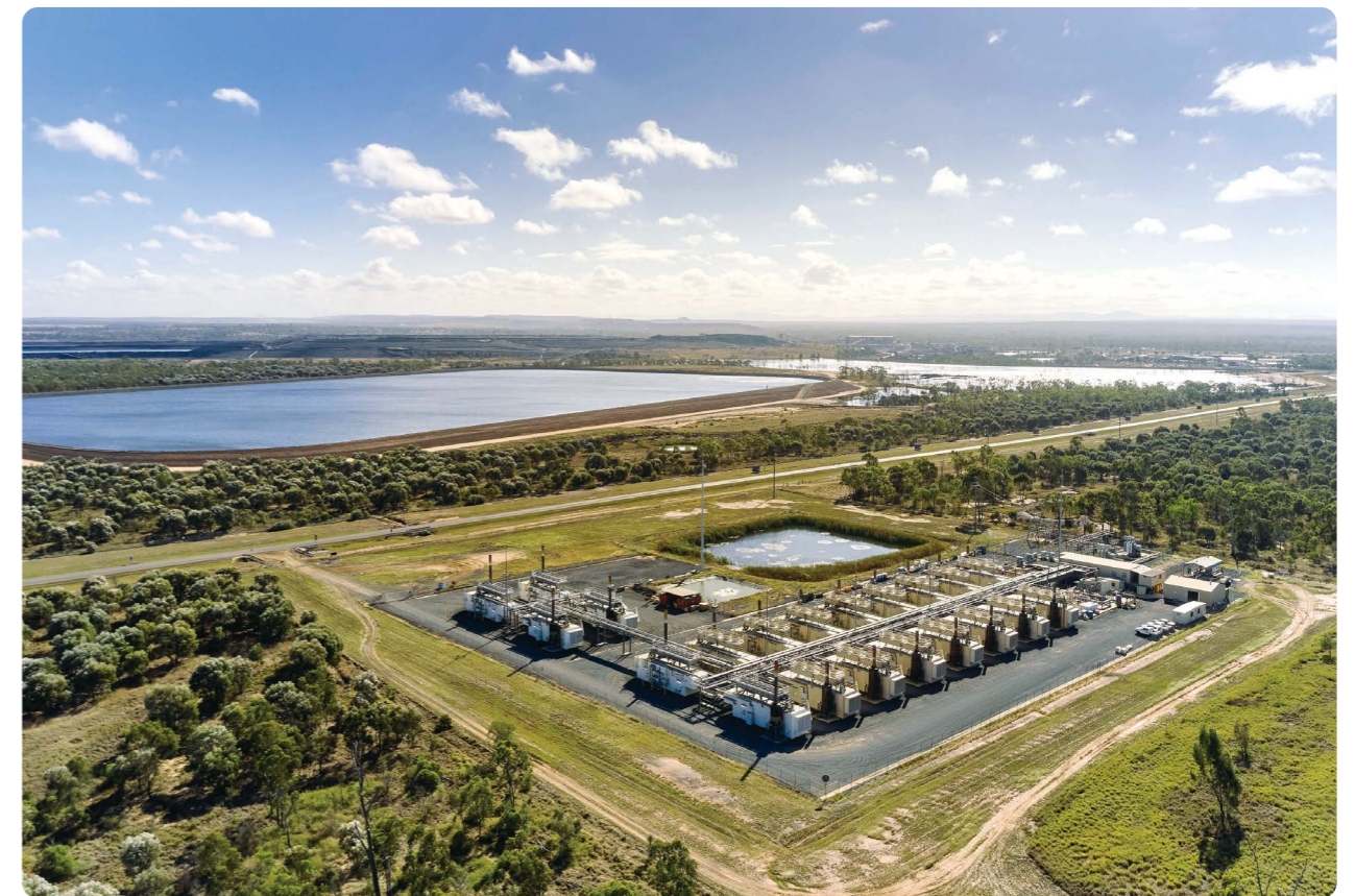
EDL owns and operates the 64 MW WCMG Moranbah North Power Station, which captures and combusts WCMG and converts it to electricity for the national electricity market.
