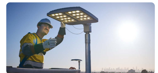
VPN’s installation of solar panel system to enhance energy efficiency.
