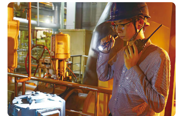
The Battery energy storage project plays a key role in maintaining a stable, reliable and good quality grid power.
