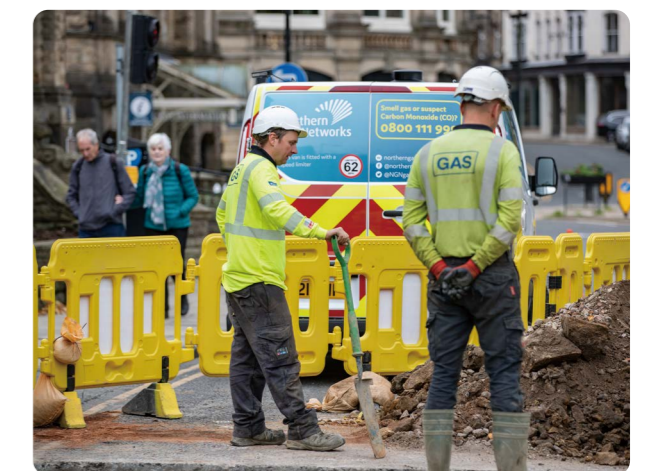
NGN engineers carry out gas mains replacement work to reinforce resilience.
