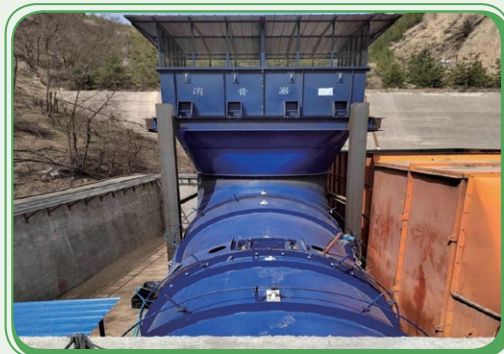
Picture: Installation of the Main Ventilation Fan
