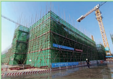
Construction Site Enclosure
