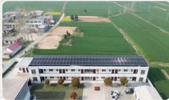
▲ Public Roof - 76kW Power Station Village Committee in Henan Province
