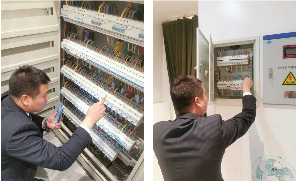
Figure: Electrical inspection
