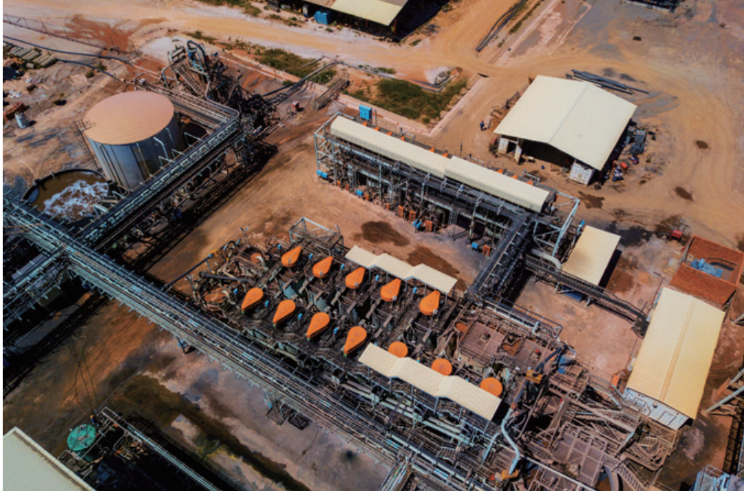
Kinsenda Processing Plant Kinsenda加工廠
