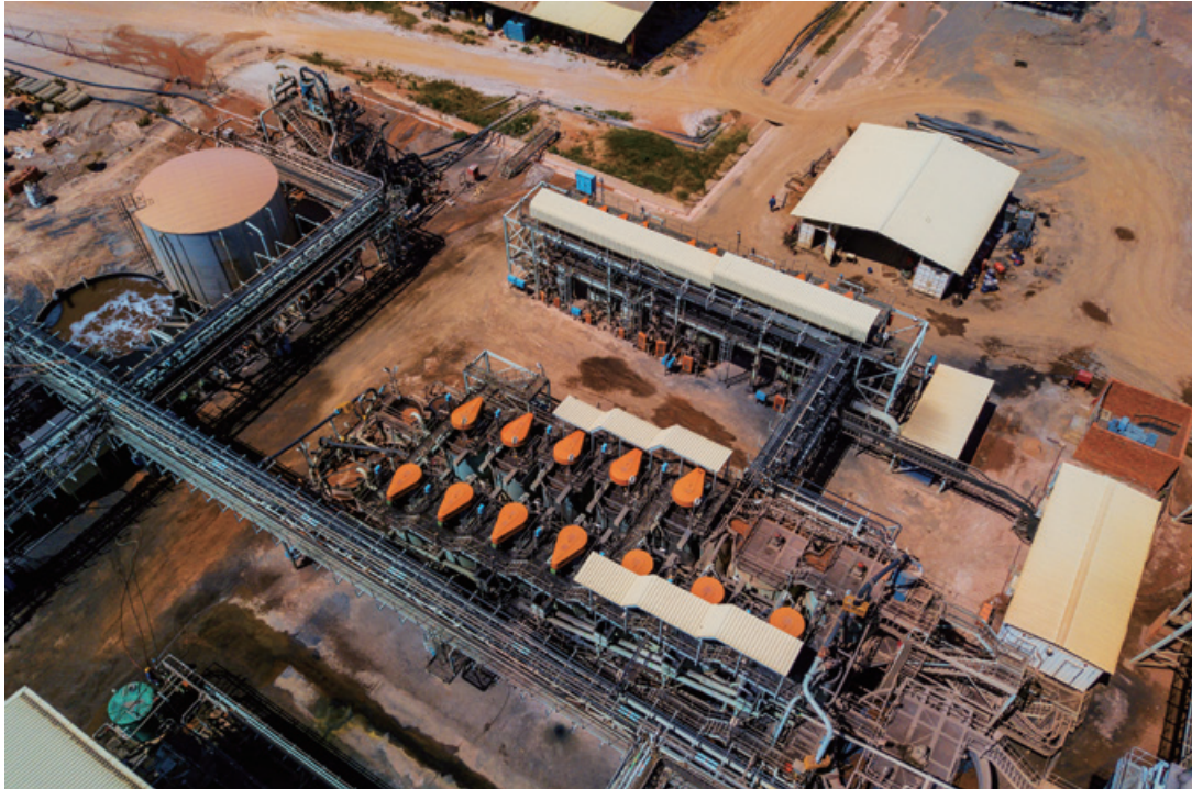
Kinsenda Processing Plant Kinsenda加工廠
