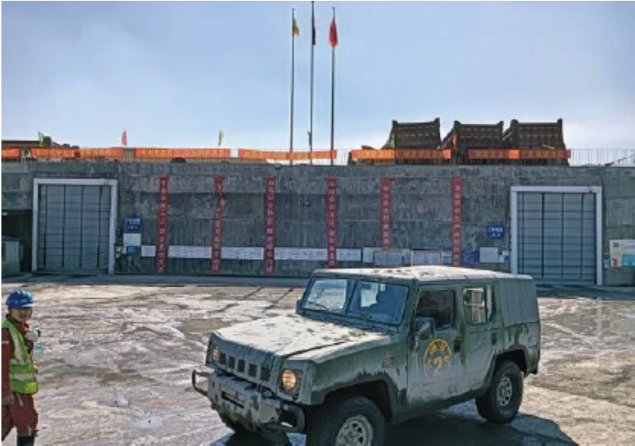
Figure 15-3 Portals to underground workings
