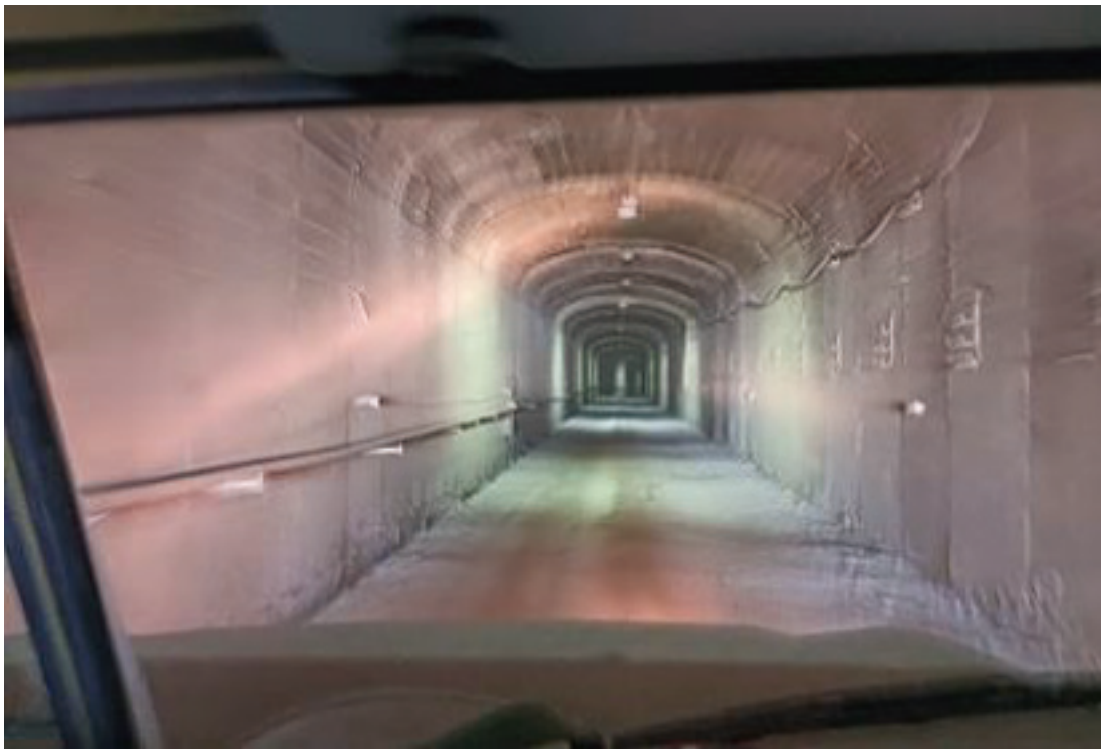
Figure 15-5 Access decline to underground workings
