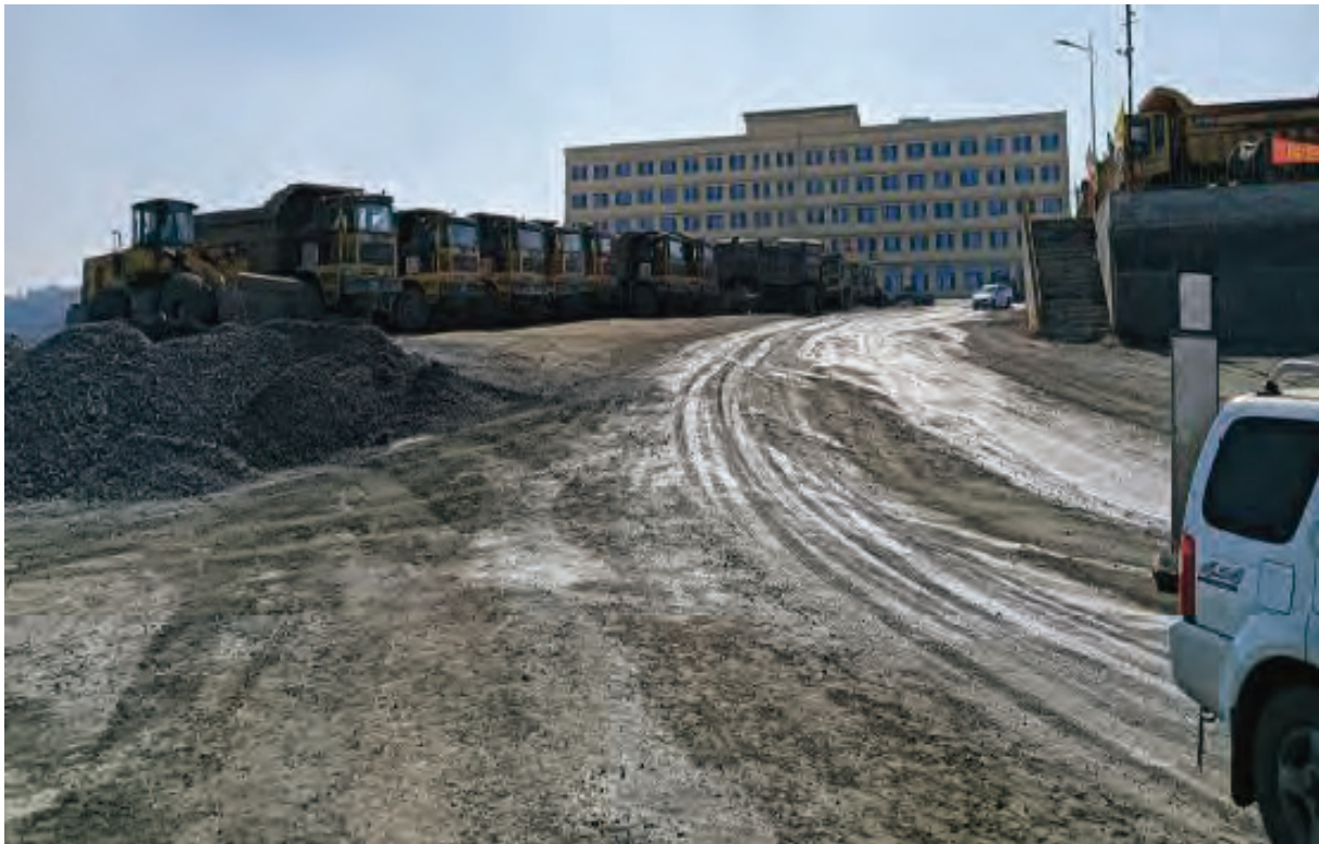
Figure 3–2 Unsealed road to site
