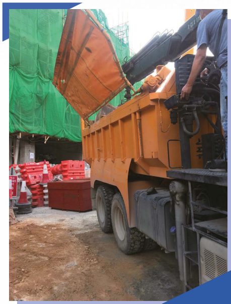
Materials covered with tarpaulin sheets 用防水布覆蓋物料
