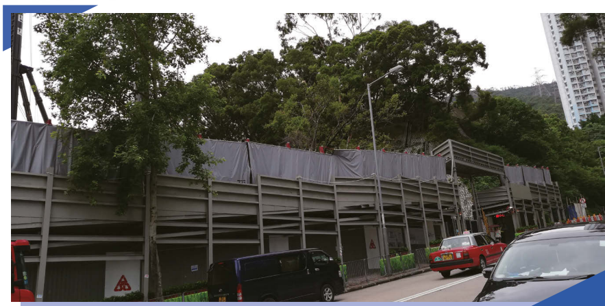
▶ Noise barriers hang on the hoarding 於圍板繫上隔音屏障
