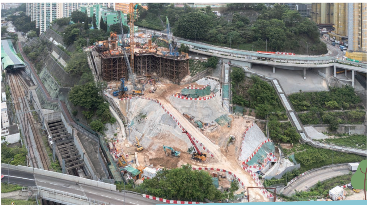
Site Formation and Foundation Works for Campus Expansion at Ho Man Tin Slope for the Hong Kong Polytechnic University 香港理工大學何文田斜坡校園擴建的地盤平整及地基工程
