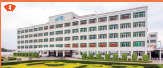
Huilai County, Guangdong Province, China
