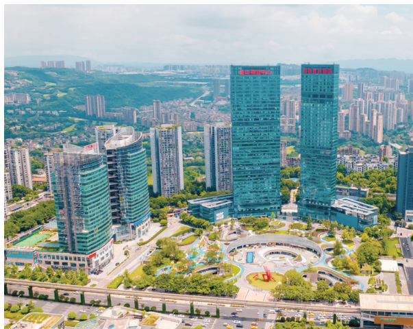
Chongqing Hon Kwok Centre and Chongqing Jinshan Shangye Zhongxin
