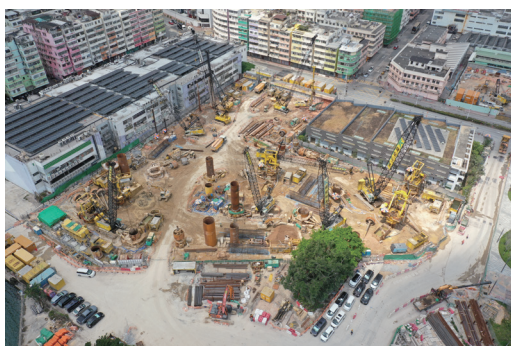
Foundation piling works at Ma Tau Kok
