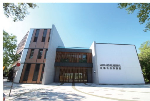
Main Contract for Peter Scott Field Studies Centre for Upgrading Mai Po Nature Reserve
