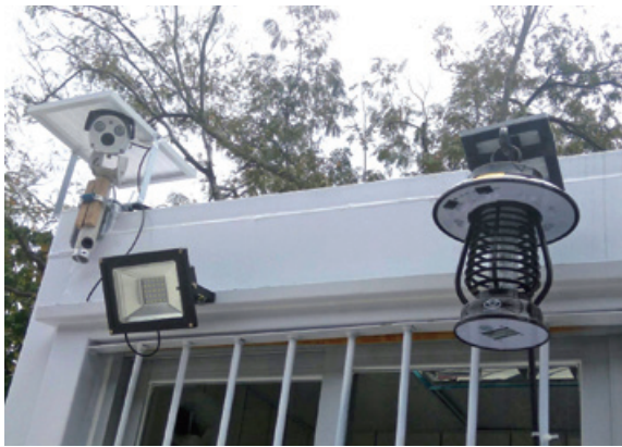
Solar powered lighting and mosquito killer
