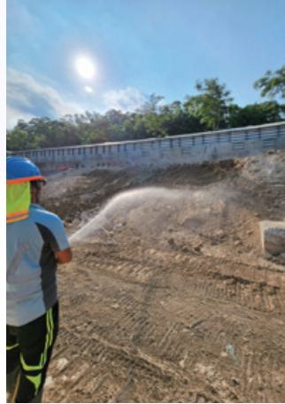
Water spraying operation to prevent dusting
