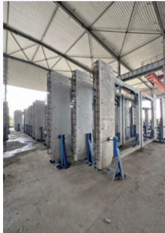
Lightweight concrete test and factory inspection
