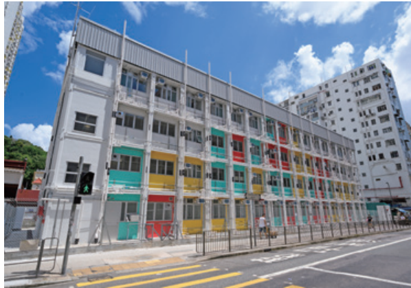
Nam Cheong 220 Project
