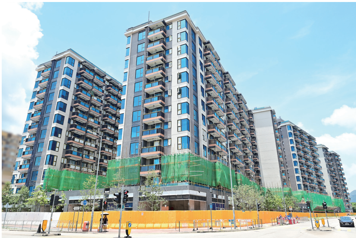
Residential development “High Park” in Hung Shui Kiu
