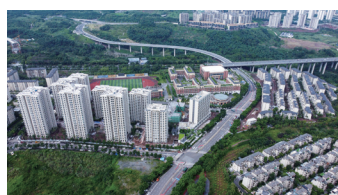
Chongqing North Star Yuelai Mansion One
