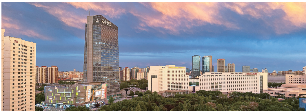
The Complex Services Building Clusters at Asian Games Village
