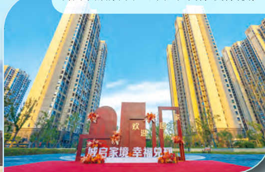
Grand delivery of CSC Zhengzhou Central Park Trio – Site view 鄭州華南城中園三組團盛大交付-交付現場2
