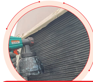
Chiller condenser before carbon film coating treatment
