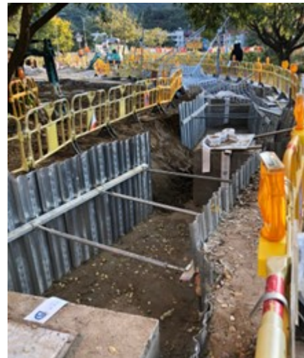
Construction of Sewage System
