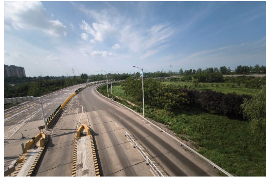
Farside View of Pinglin Expressway
