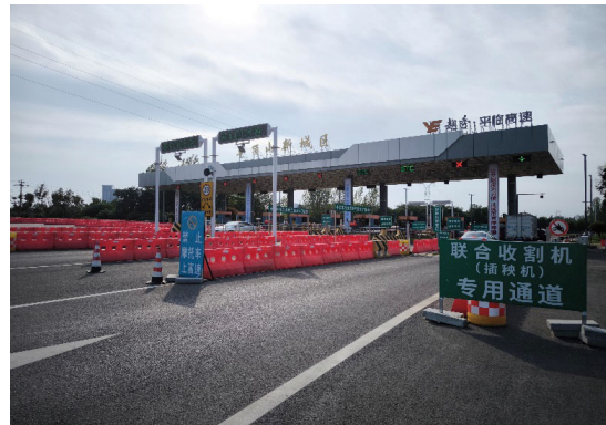
Pingdingshan City Toll Station
