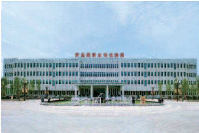
Photo: Our production facility in Changle county, Weifang, Shandong Province, the PRC
